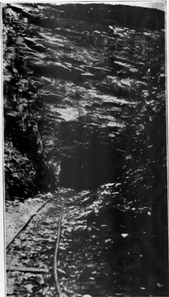
Entrance to Tunnel
